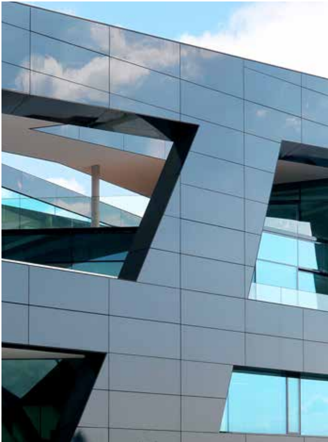
Transition from the black, non-visibly fixed glass elements with open joint pattern to the reveals
