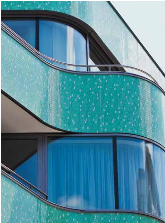
Detail view of the curved facade strips with glass mosaic cladding
