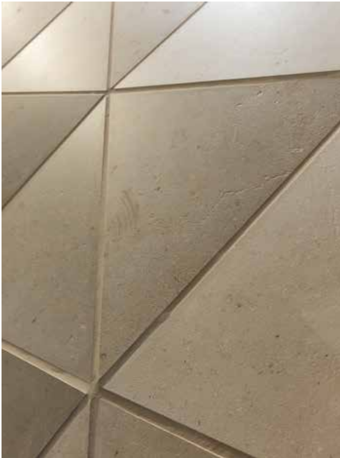
Detail view of natural stone tiles as perfectly cut-to-size cladding for individual shapes, tinted pointing mortar as an additional design element
