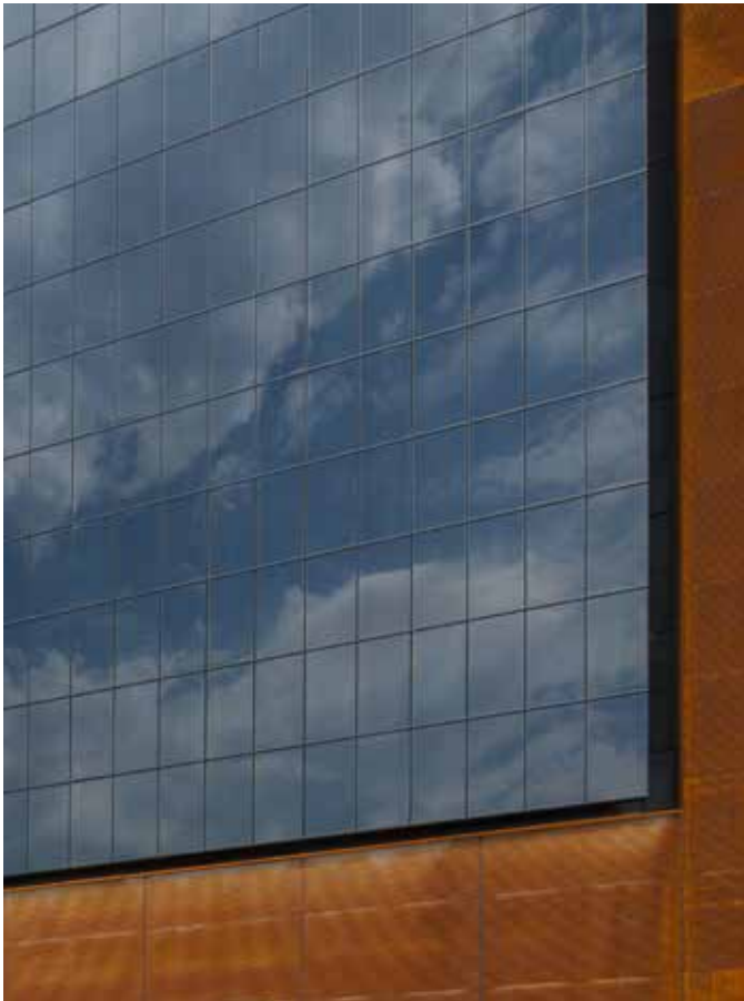
Detail view of the framed photovoltaic facade elements
