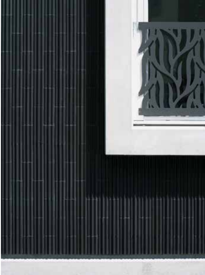
Material transition from plinth and window to the ceramic facade
