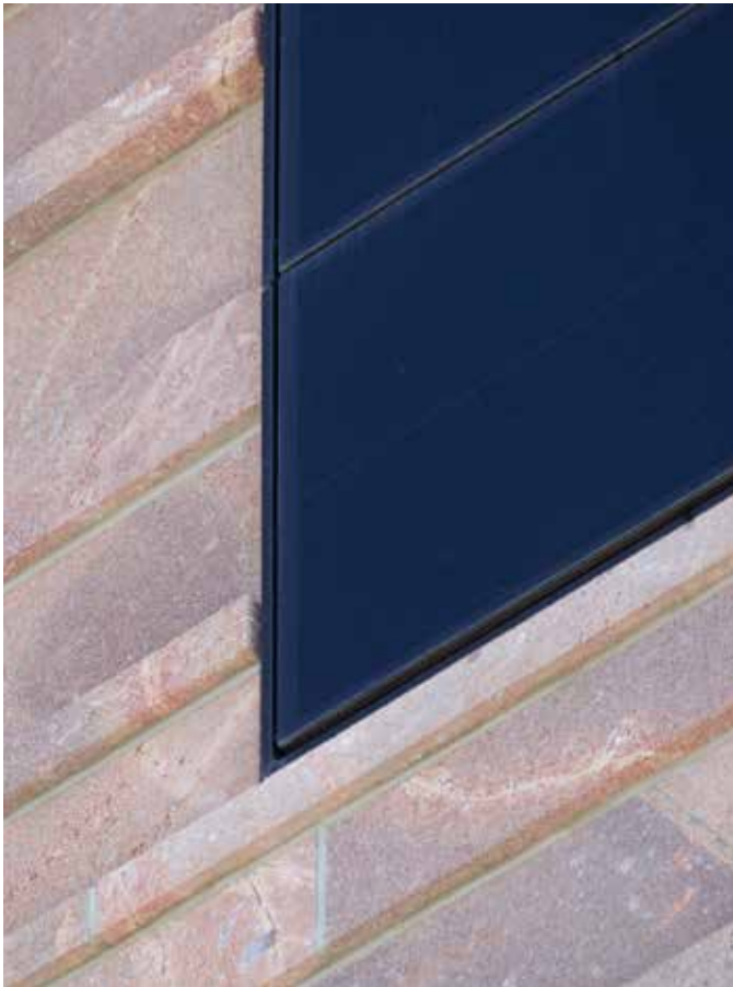
Detail view of the transition between the non-visibly fixed photovoltaic panels and the natural stone facade
